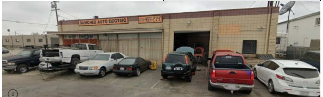
View of east side of the building
