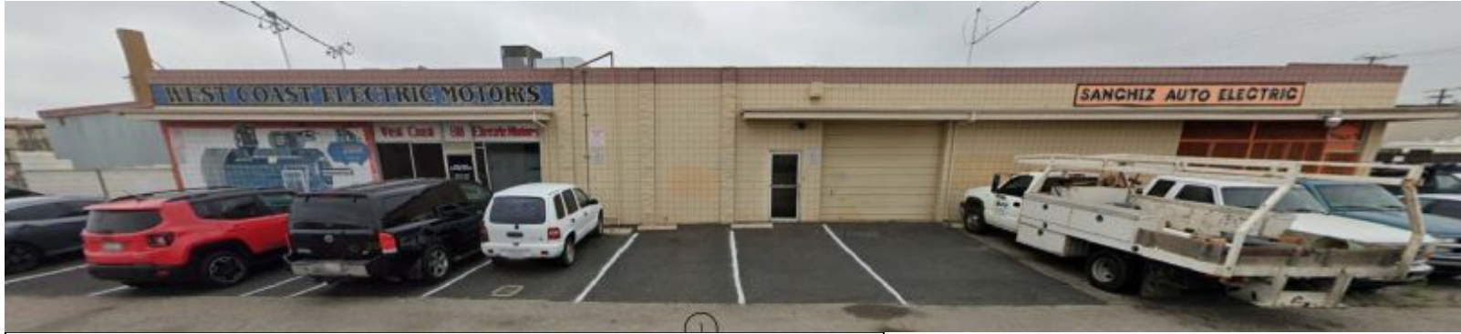
From Mercantile looking north at the front of the building
