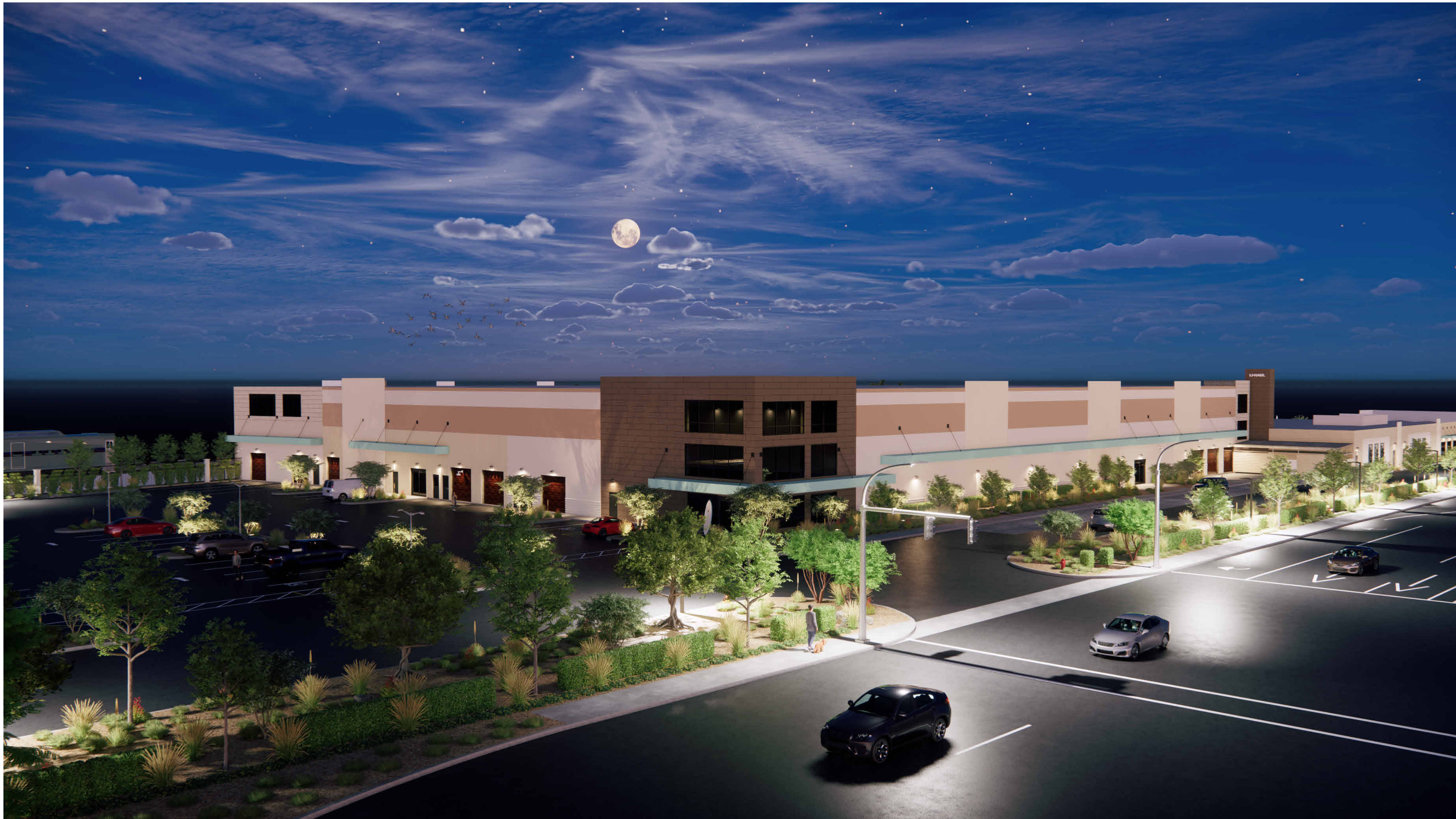
AERIAL VIEW NIGHT TIME
