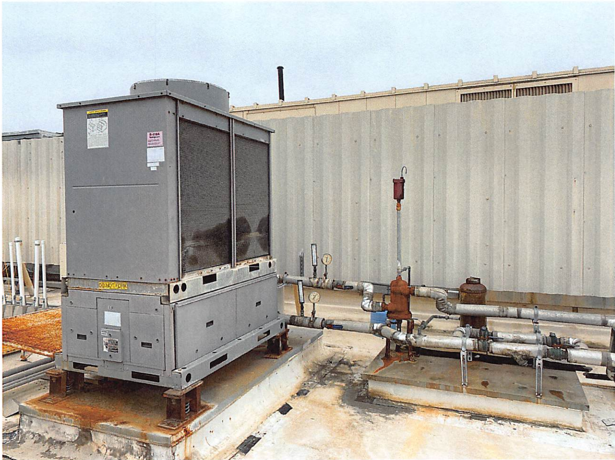
Roof Top Exterior
