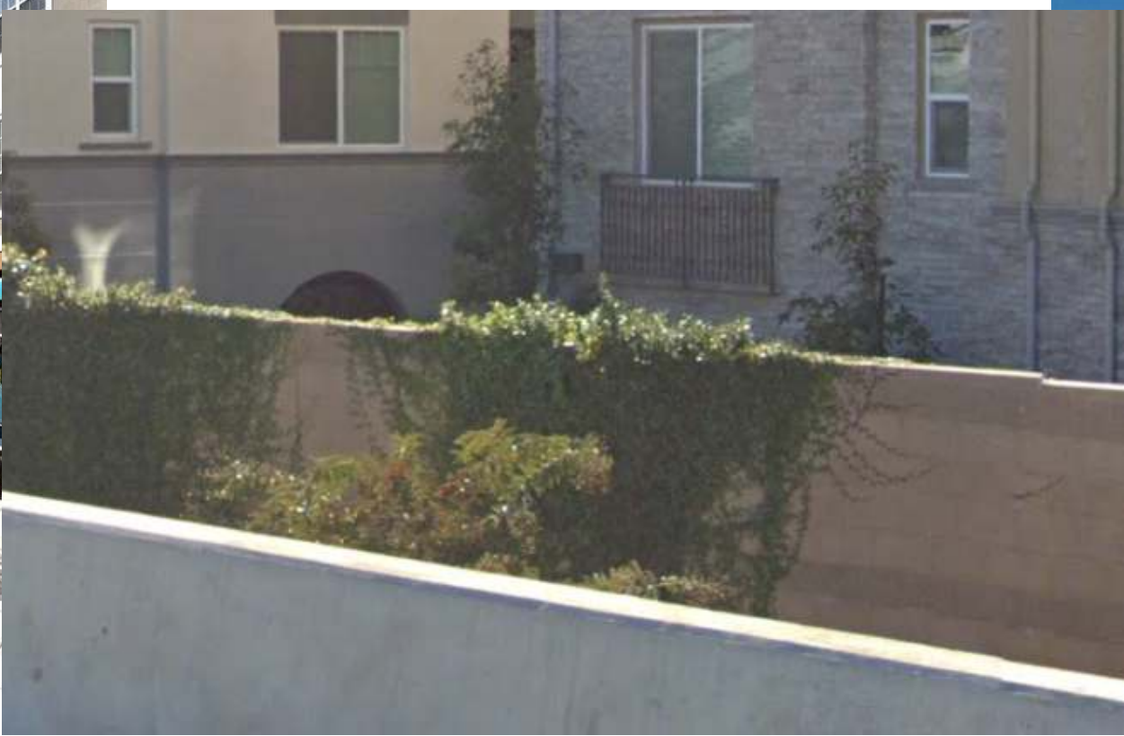
FREEWAY SCREEN WALL (AT WAGON WHEEL ALONG FREEWAY)
