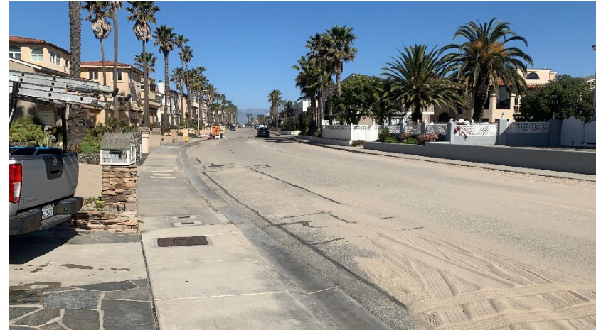
Photograph 2. View of Sand Removal Area 2, between Seabreeze Way and Neptune Square, facing south.
