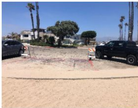
Photograph 17. View of sand removal area at Channel View parking lot in Area Five.
