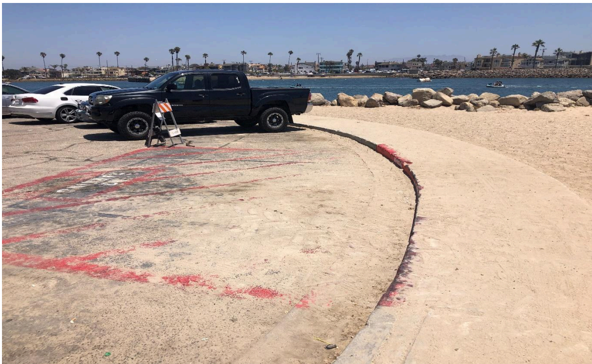
Photograph 14. View of sand removal site at Channel View Park (aspect east; July 20, 2021).
