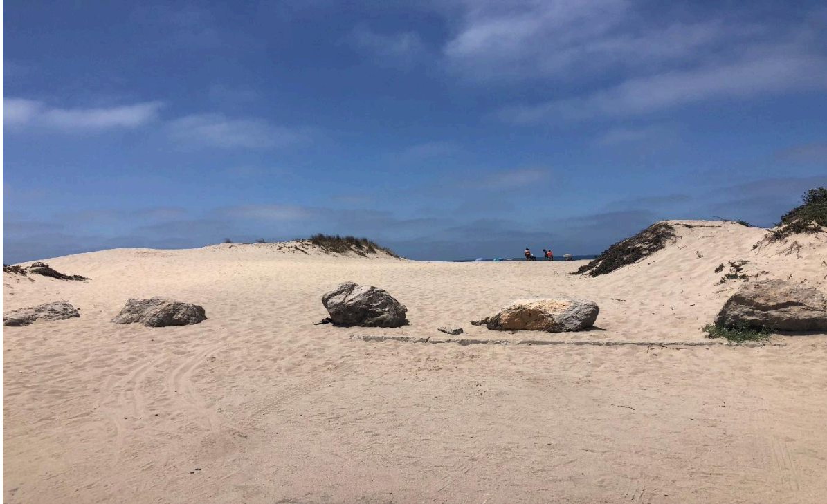
Photograph 13. View of access, sand removal and work area at Oxnard Shores parking lot (aspect west; July 20, 2021).
