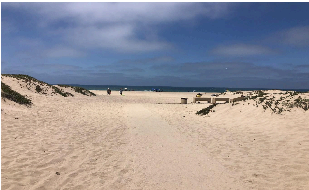
Photograph 12. View of work area and sand placement site west of Oxnard Shores parking lot (aspect west; July 20, 2021).
