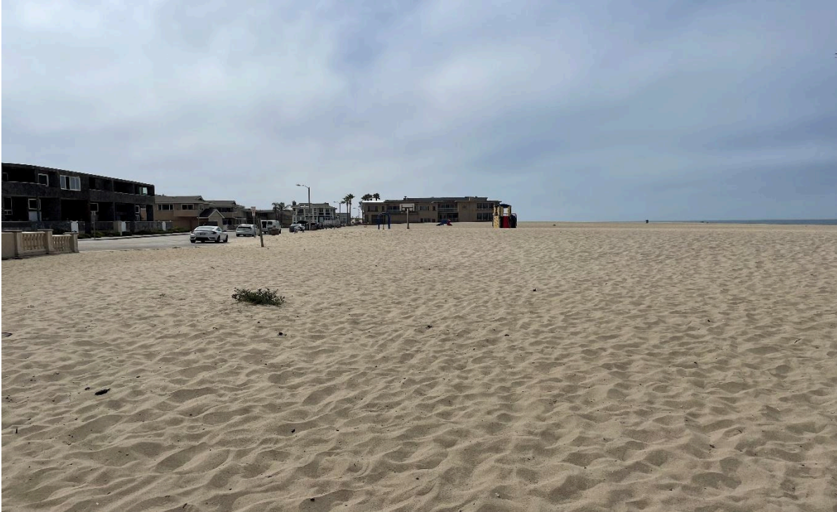
Photograph 5. View of sand placement and work area at Neptune Square (aspect south; July 20, 2021).
